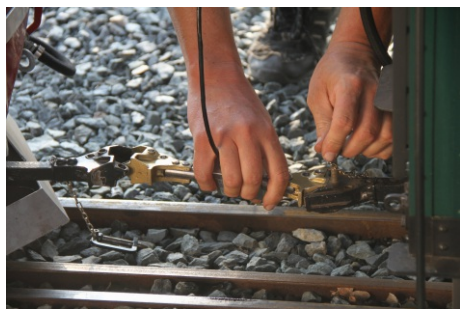
Instalace do vlaku
